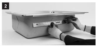
Take a ruler or straight edge and trace a line on the underside of the sink where you would like the BOTTOM of the SinkMate backing strip to be placed, keeping the line level to the top of the sink.
