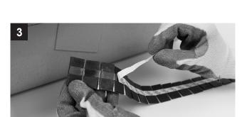
Clean surface of any loose sound deadening, grease or dirt. Remove packaging from SinkMate backing strip. Peel back the double-sided tape as shown.
